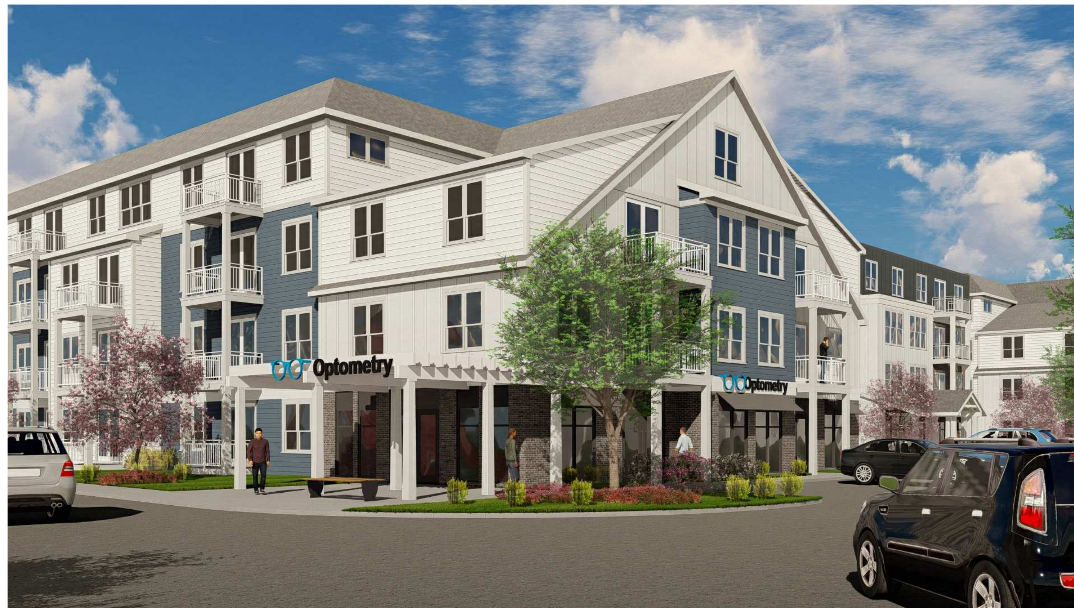
VIEW FROM POND STREET - COMMERCIAL
